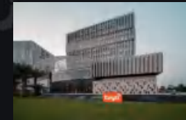
Hangzhou China HQ-Hangzhou Tuya Information Technology Co.,Ltd
